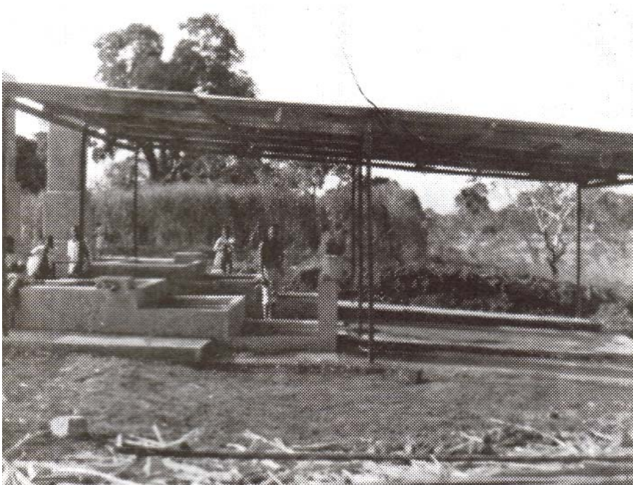
Figure A2: Photograph of Evaporators
