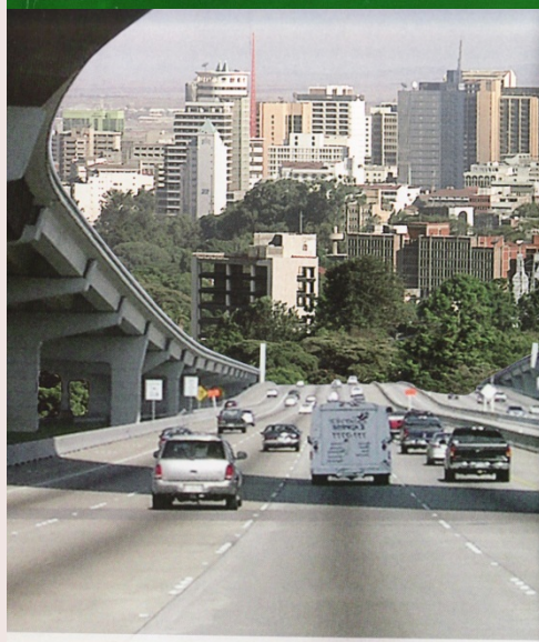
City of Nairobi in the future: the 2030 Vision aspires to a capital firmly interconnected through a network of roads, railways, ports, airports, waterways and telecommunications.
