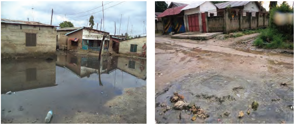
Figure 6.3: Sewerage inadequacy in Kawe Mzimuni
